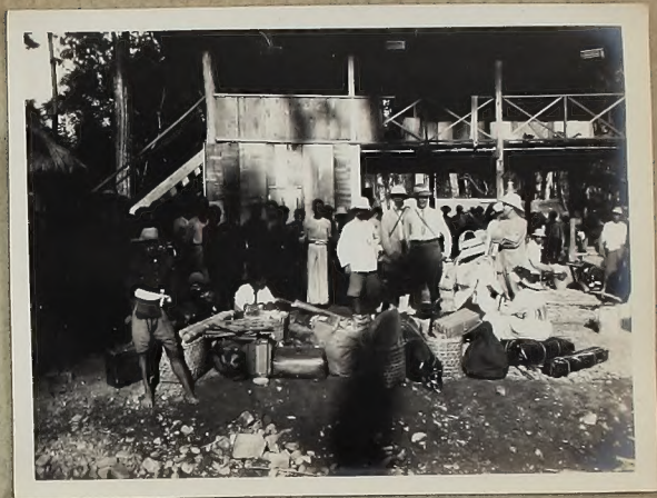
Pak. Kahi - waiting for the construction train & Road built in jungle of Western Borneo
